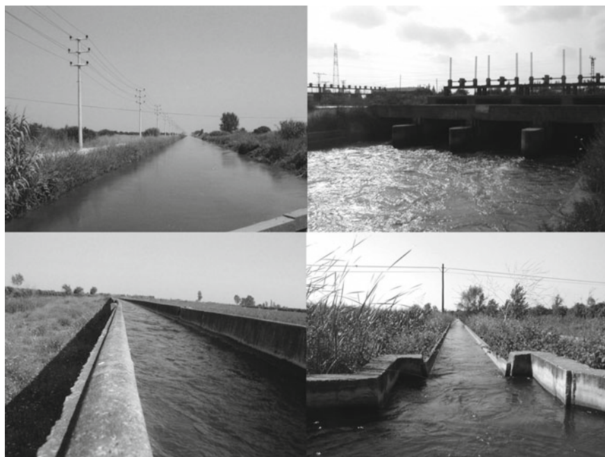
Fig. 15.3 Irrigation facilities in the Lower Seyhan Irrigation Project (Top left: Conveyance canal; Top right: Diversion weir; Bottom left: Secondary canal; Bottom right: Tertiary canal). Source Photos by Chieko Umetsu
